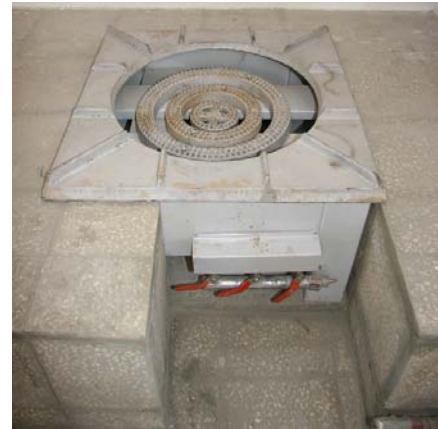
Figure 5 - The propane stove dropped into the concrete platform.
