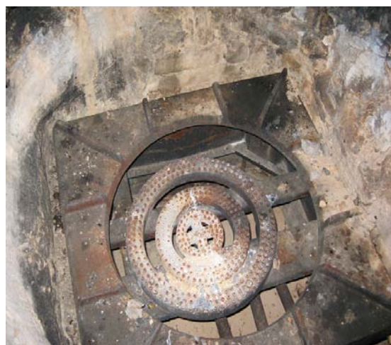
Figure 2 - Legacy Converted Propane Stove (set into the firebox and not accessible for cleaning and replacement)
