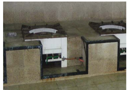
Figure 6 - The propane stove dropped into the concrete platform.
