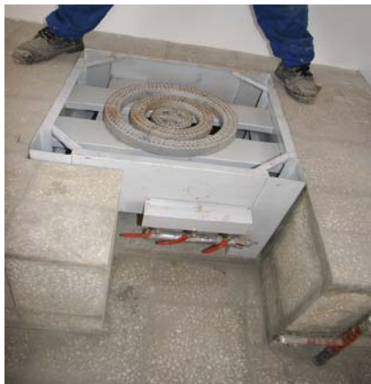
Figure 4 - The propane stove dropped into the concrete platform.
